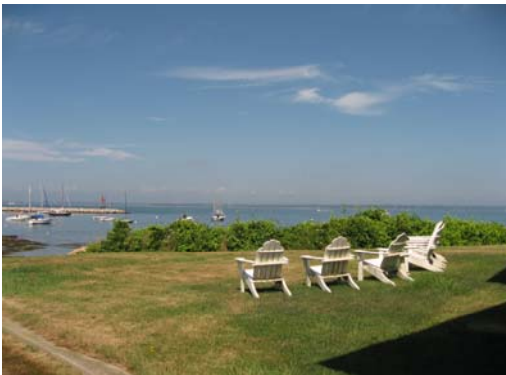
Looking west to the Sakonnet breakwater
